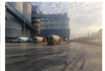
Enclosed Bulk Cement Dispatch
