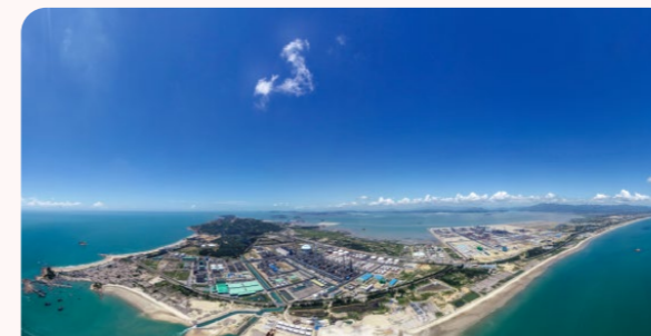
SABIC Fujian Petrochemical Ethylene Project Site in Gulei
