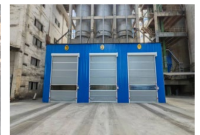
Enclosed Clinker Dispatch
