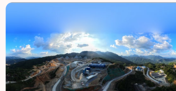
Mulan Pumped Storage
