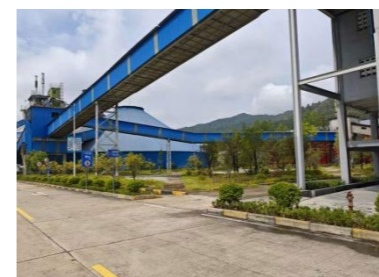
Enclosed Material Conveying Corridor
