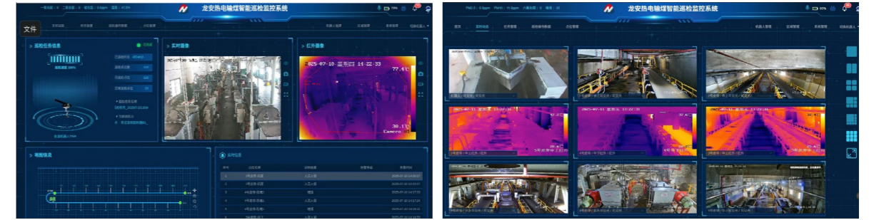
Long'an Cogeneration Power Intelligent System
